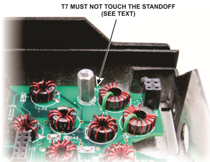
Figure 36. Checking T7 Clearance.
